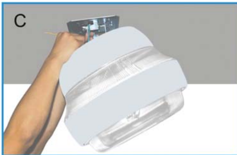
With hands free, make electrical connections
